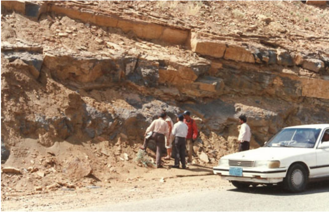
Fig. 3.37 The picture shows a slab slide on a hill road in Yemen. Parking of car right at the site and work at the site without helmets are bad practices which must be avoided
