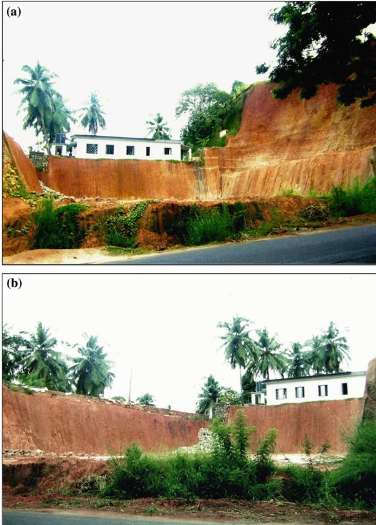
Fig. 3.51 a and b The two pictures of a high, unsupported cutting in residual soil formed by in-place weathering of basaltic rocks is from the city of Mangalore in the State of Karnataka in India. The common observation that fairly deep cuttings can stand vertical without outer support encourages building contractors to make such cuttings when needed, even very close to the existing buildings, as shown above. They ignore the fact that a cutting which is safe today may fail tomorrow or after a few years. Why should a cutting which is safe today should fail subsequently? It is the question we must answer. (Photos Ashok Mendonca)
