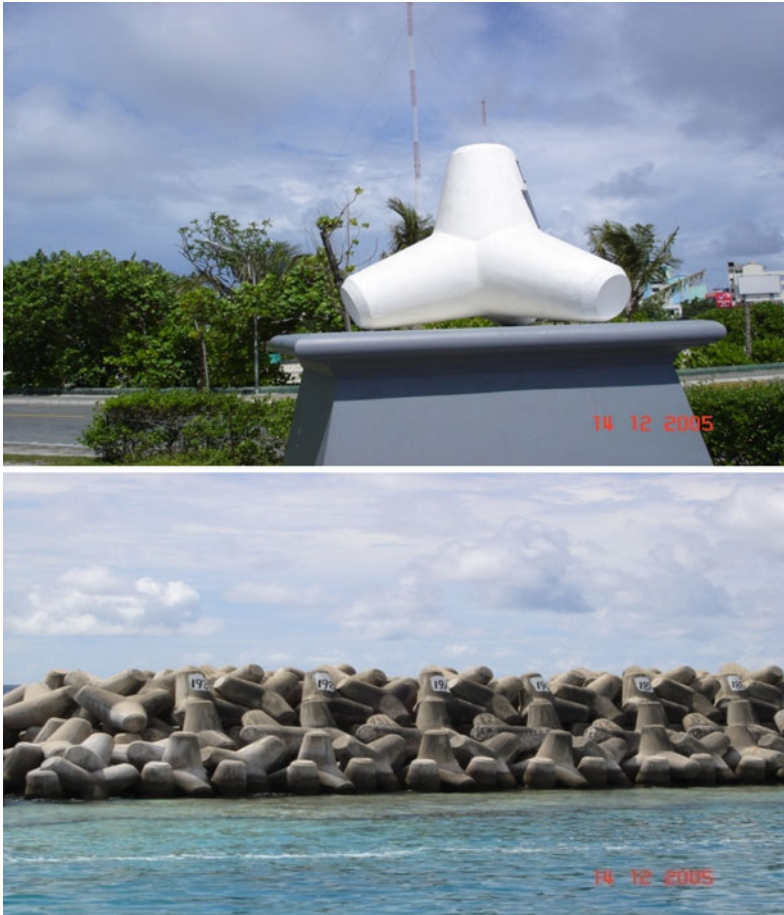
Fig. 3.71 The use of tetrapods for the protection of water bodies, river banks, and coastal belts against tidal waves and water forces has a great advantage over the use of reinforced cement concrete (RCC) cubical blocks because of their unique shape and inherent stability. Unlike the RCC blocks, tetrapods respond to erosion, sinking, and water forces in a manner that they maintain their stability at all times. The above pictures taken by the author are from Maldives which offer a good example of coastal protection by tetrapods. It is usual to number the tetrapods for tracking their locations at any given point on time
