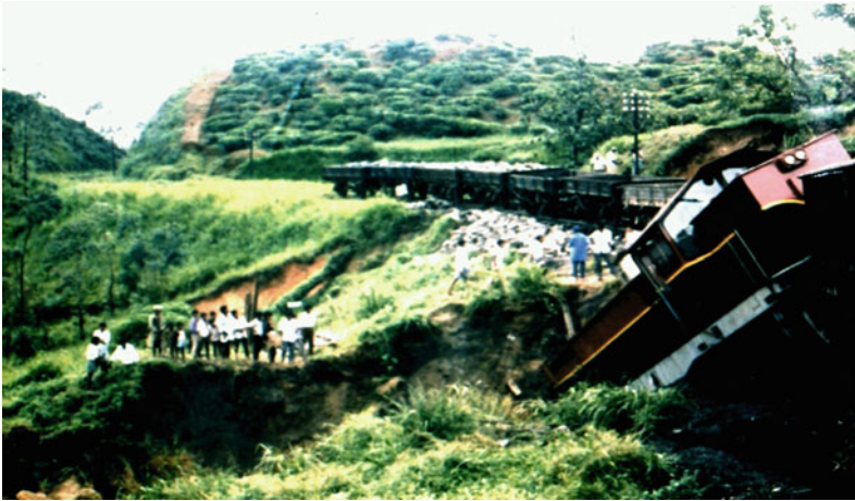
Fig. 8.28 The above picture is of the famous Watawala earthslide in Sri Lanka which affected a railway line for decades on end. On 3 June 1992, at about 5 a.m., the engine of the Hatton–Colombo goods train nose-dived and sunk disrupting the train services. Scarcely 1 h before this accident, had the Colombo–Badulla passenger train with 3,000 passengers passed the very same location
