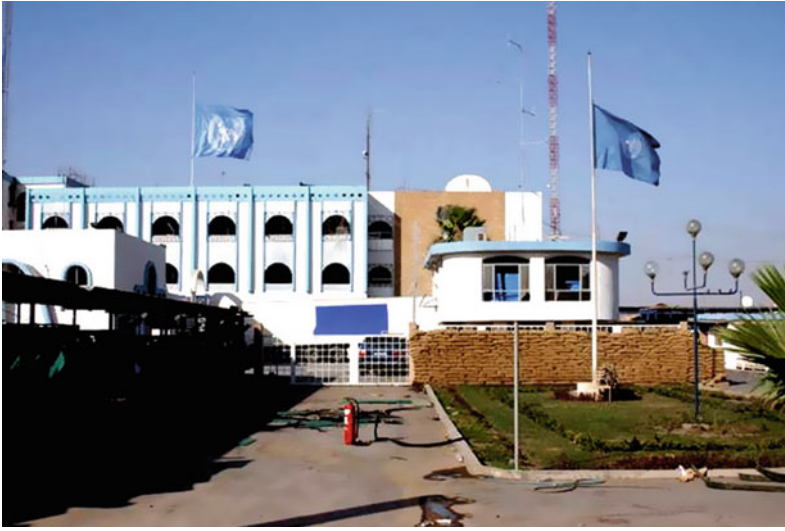
Fig. 5.3 The UN building in Baghdad before the terrorist bombing of 19 August 2003 in which 19 United Nations staff including the special representative of the U.N. Secretary General were killed. The author was a member of the UN team in Iraq at that time
