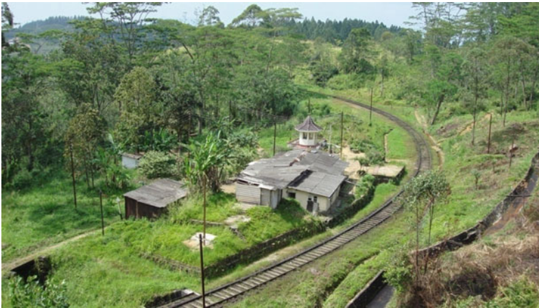
Fig. 8.29 The Watawala earthslide considered intractable in 1992 was fixed in 1995 jointly by the National Building Research Organization, Colombo, the Sri Lankan Railways, and UN-HABITAT taking recourse to one of the most carefully conducted scientific studies. The earthslide was stabilized using the technology of direction drilling to create a network of long and continuous self-actuated subsurface drains. So successful was the remediation program that Watawala earthslide is a history now
