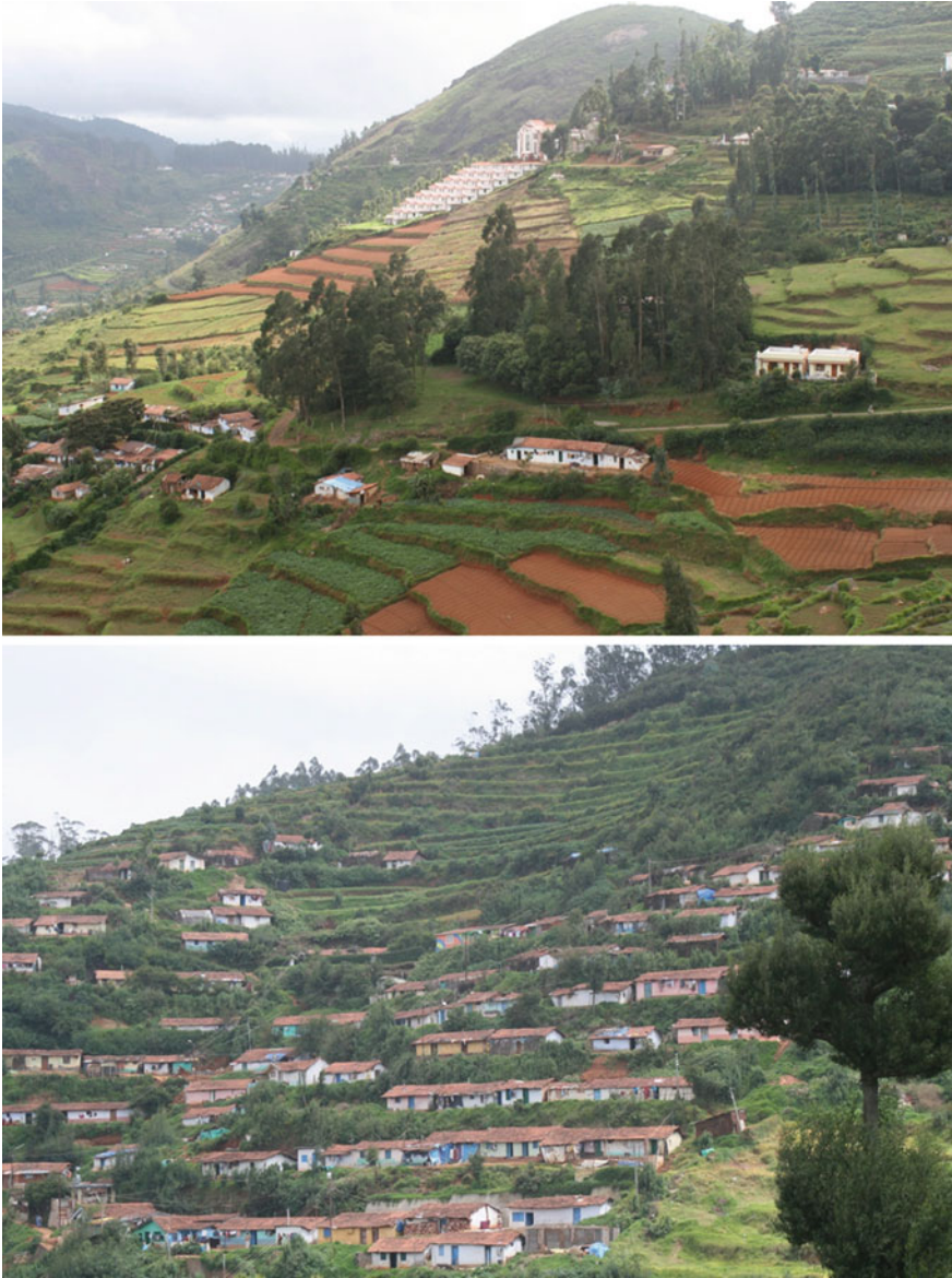
Fig. 8.26 The above pictures show examples of engineered townships against landslides. Planning of housing layout, use of design codes of practice, minimization of violence against slopes, protection of its vegetative cover and caring for its surface and subsurface drainage are some of the design features. The slope behavior will now depend on its drainage and maintenance
