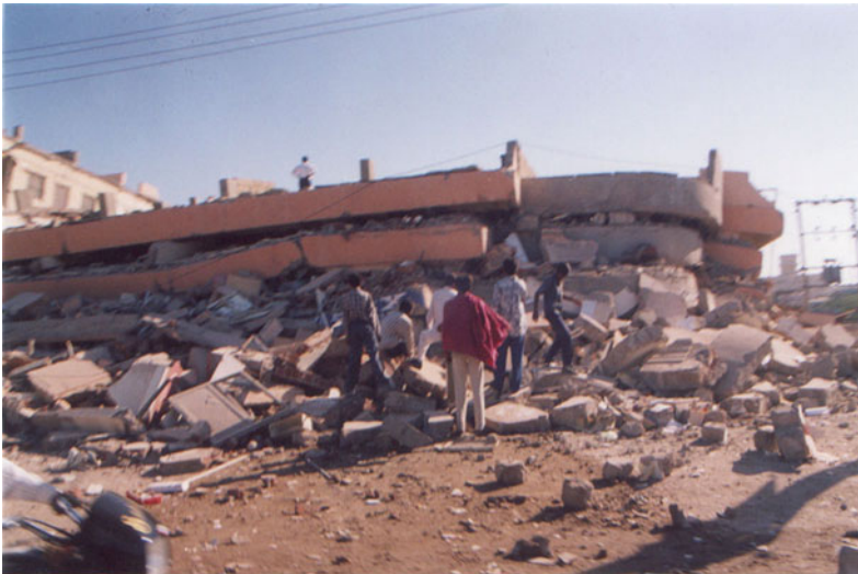
Fig. 3.17 View of a building in Gandhidham, Gujarat which collapsed like a deck of cards during the earthquake of 26 January 2001. This type of building collapse is typical of building failures due to the loss of support between the floors
